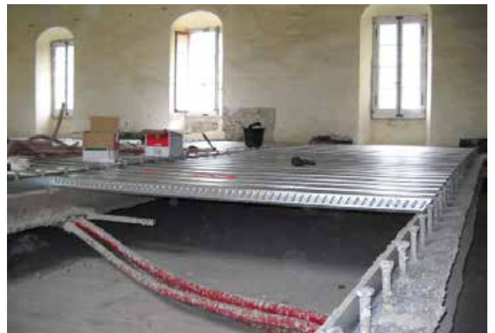
Installation within rehabilitation project - Cofraplus® 60
