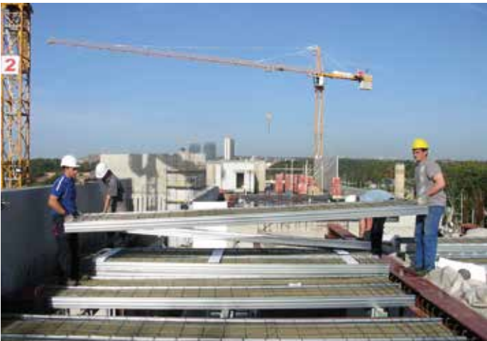
Installation of Cofradal® 200
