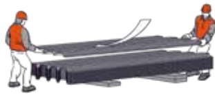
11 ■ Handle profile sheets correctly
