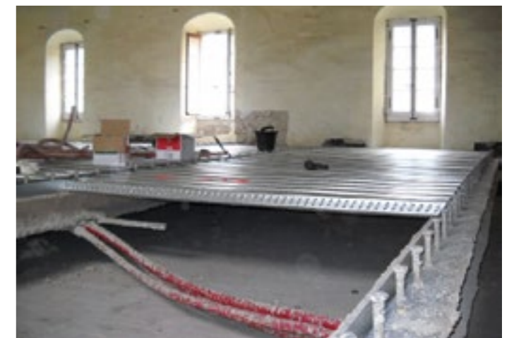
Installation within rehabilitation project - Cofraplus® 60
