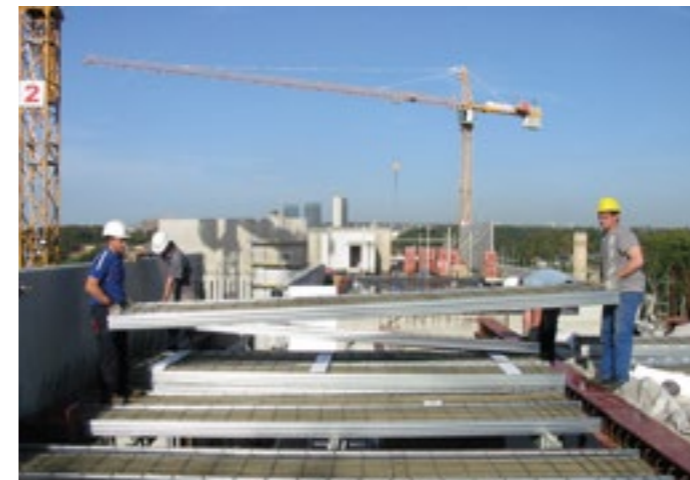
Installation of Cofradal® 200
