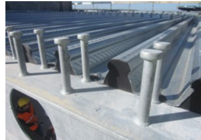
Cofrastra® 70 with profile filler installed on composite beam with double shear studs
