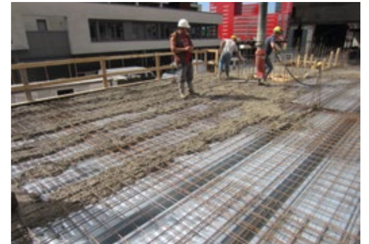
Concrete pouring on Cofraplus® 220 filling first the ribs
